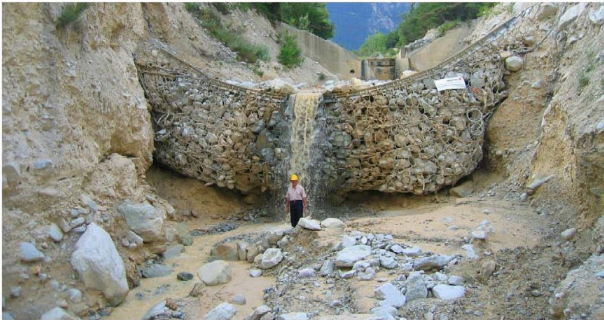
Figure 4. Landslip stopped by high-strength steel fence
